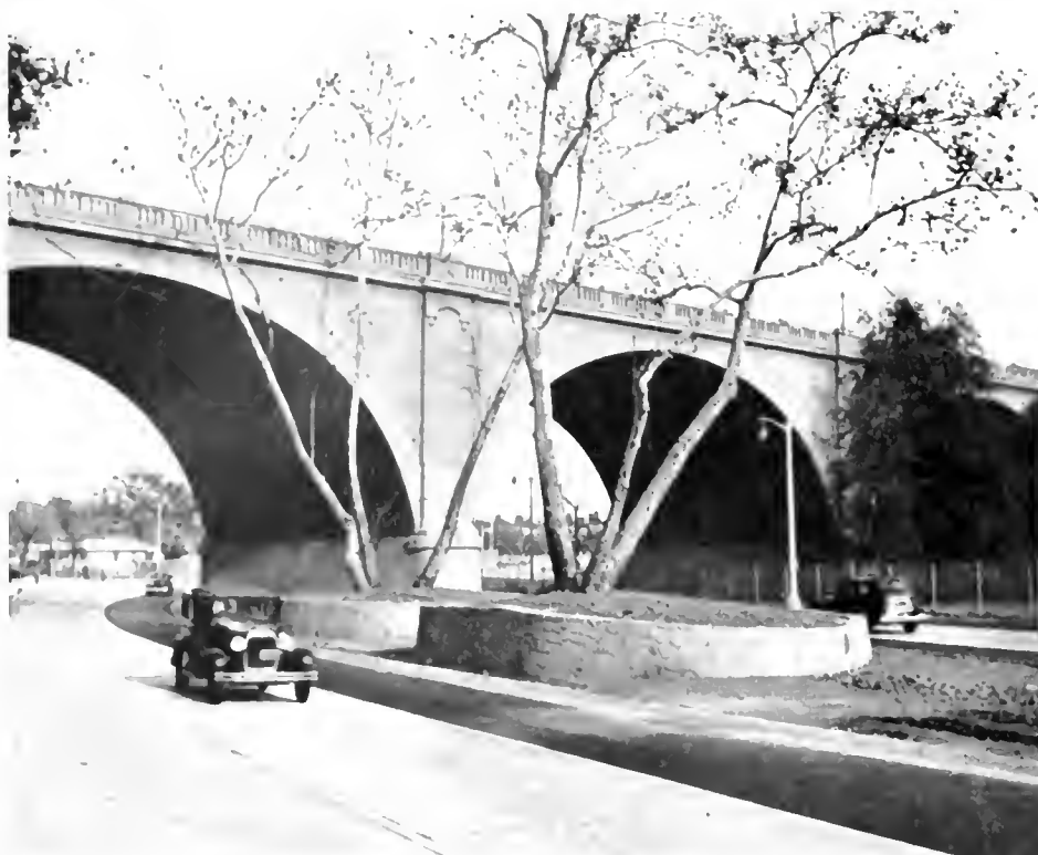
Great care was taken to protect natural sycamores with masonry retaining walls
